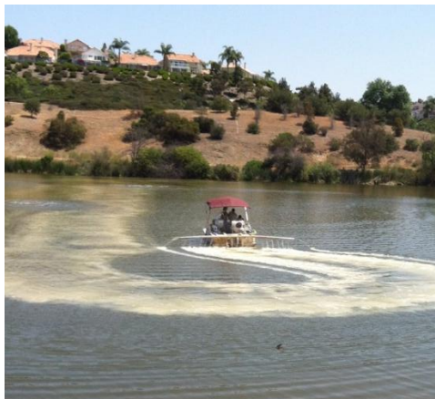
Figures 2 & 3: Phoslock application to 4 established zones of Laguna Niguel Lake.
