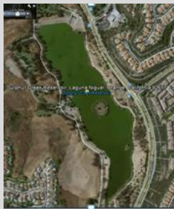
Figure 1: Aerial view of Laguna Niguel Lake (2009)
