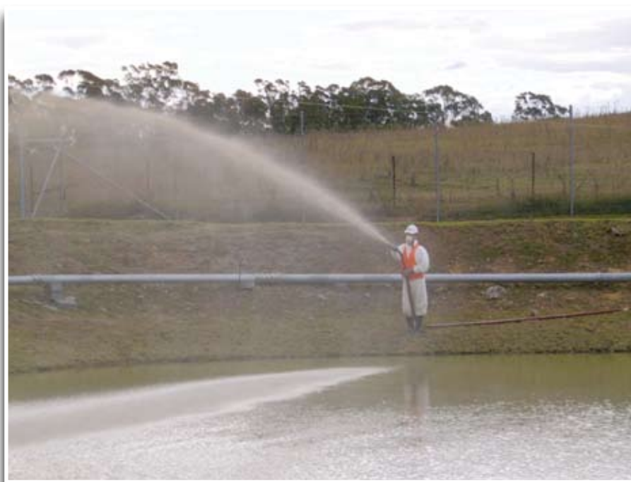
Phoslock application for treatment of recycled water ponds
